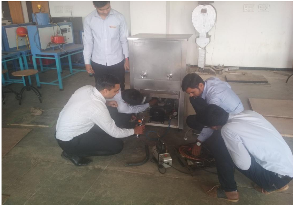
Gas Charging & Brazing of copper tube
