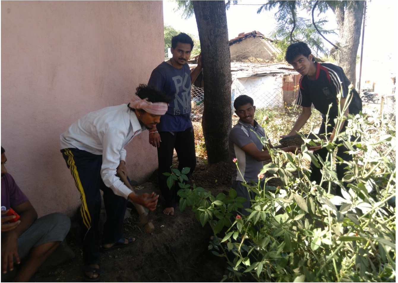
Digging of Soak Pits at Savargaon during NSS Camp
