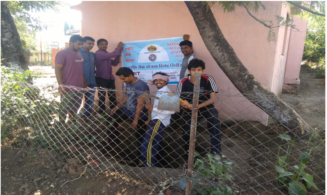
Digging of Soak Pit in School Premises (Savargaon Village)
