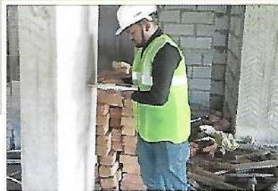
Rebound Hammer test
